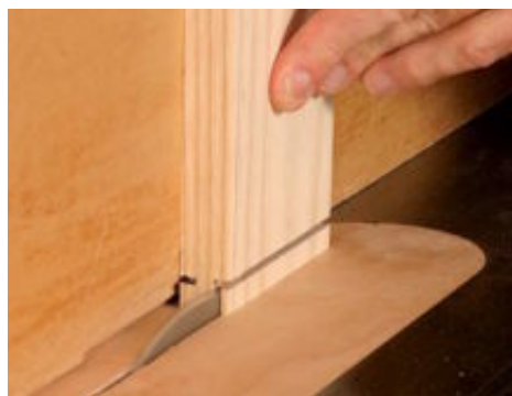
Cut the stub tenons. Raise the tablesaw blade enough to barely nick the bottom corner of the groove (top). This ensures a clean, snug-fitting corner at the base of the tenon. Raise the blade to trim the tenon cheeks (bottom).
