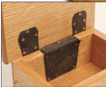
Leather. Three pieces of leather—two end pieces and a center piece—are secured with brass tacks to create a unique hinge.
