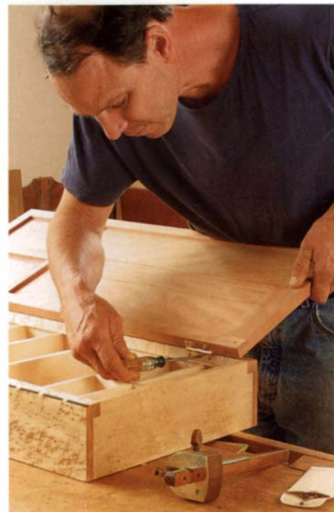
Installing butt hinges, p. 52
