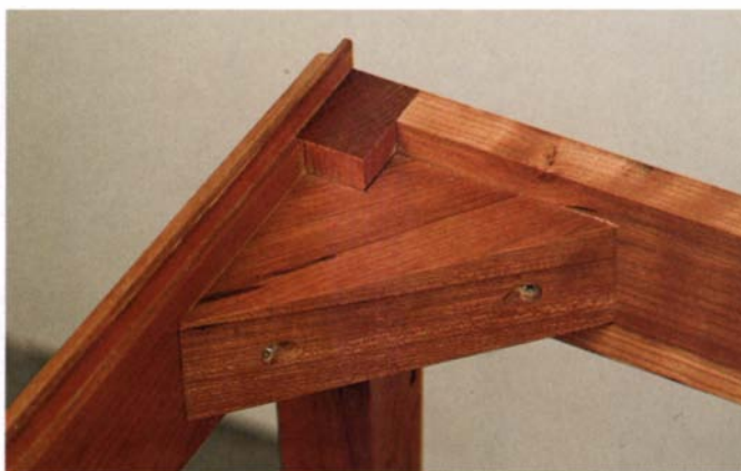
Supporting heavy loads —Corner braces reinforce the mortised-and-tenoned rail-to-leg joint and enable this elegant base to support the heavy tool chest.
