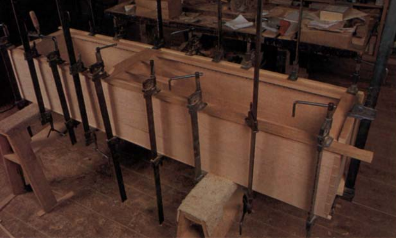
During glue-up, clamping strips are used to protect the face frame and the rabbet on the back edge. The large number of clamps ensures a good bond. The wedges and batten help secure the center-frame rail, where clamps won't reach. Wedges under the feet of the sawhorse remove twist from the carcass.
