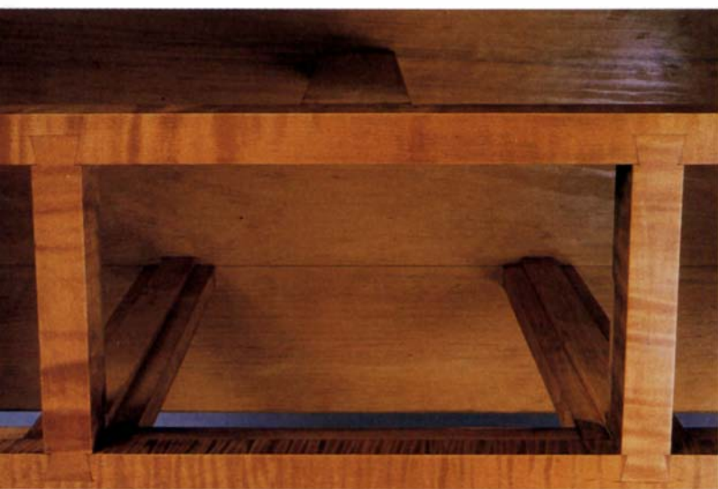
The central drawer runners are mortised into the back of the carcase and rest on a cleat nailed to the back of the front apron. A brace mortised into the back of the carcase and into the middle horizontal divider keeps this drawer from tipping when opened.
