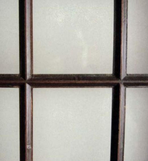
A multi-paned glass door dresses up the author's walnut corner cabinet. Detail at left shows how crisp putty lines define inside surface of the glazing. The putty is tinted to match the wood.
