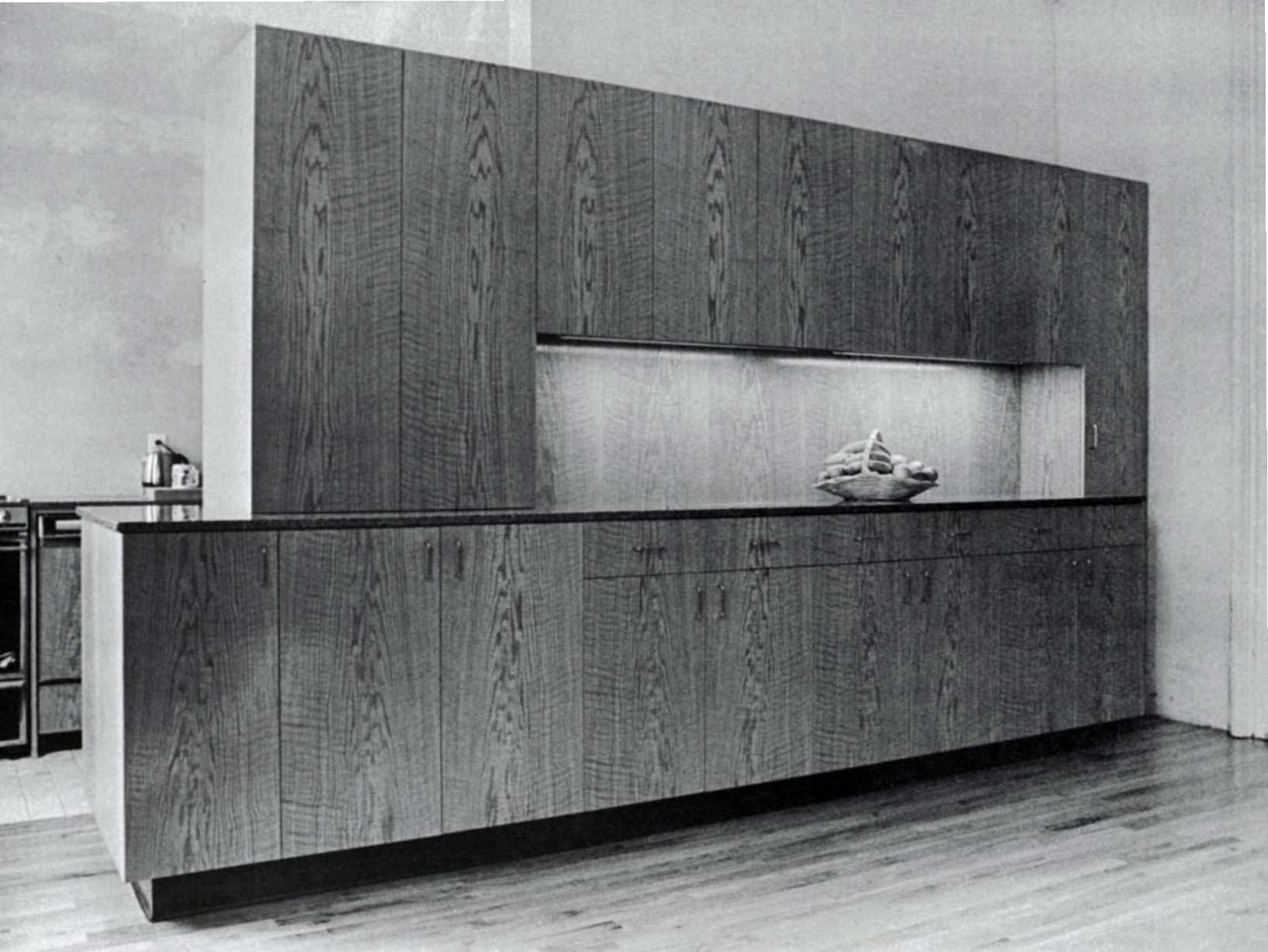
Bookmatched doors hinged on concealed hardware make for clean, uninterrupted kitchen cabinets.
