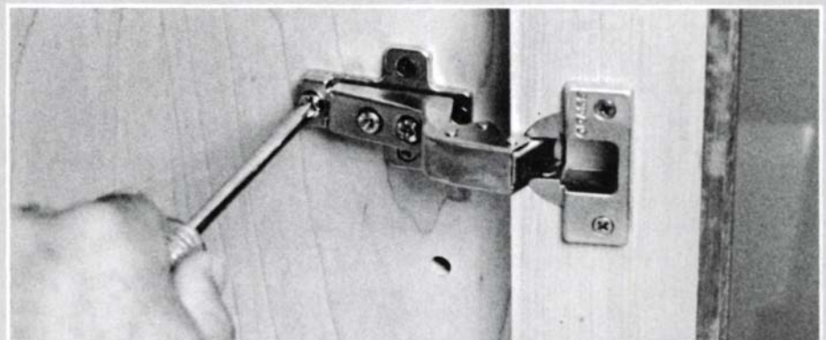
In the arm of this hinge, the screw at the right controls the door's lateral position; the middle screw, its distance from the front edge of the carcass. The third screw, when loosened, allows the door to be moved up or down in the vertical plane.
